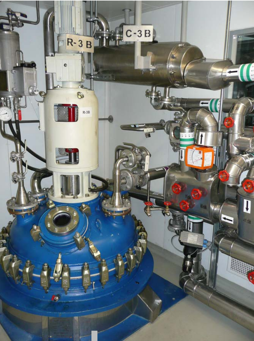
650-L reactor in grey controlled area
